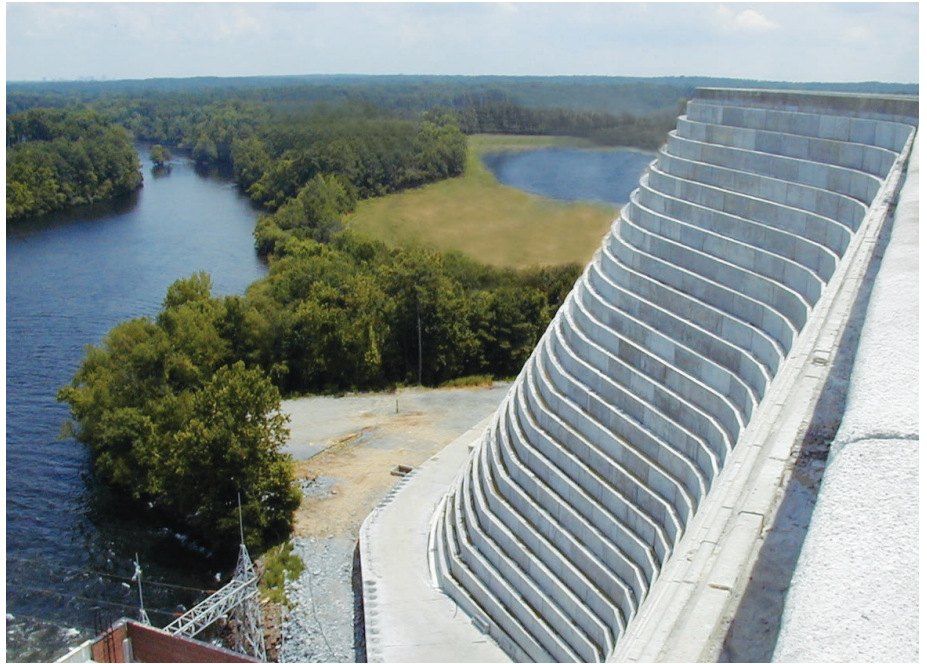
Lake Murray Dam Project in South Carolina
